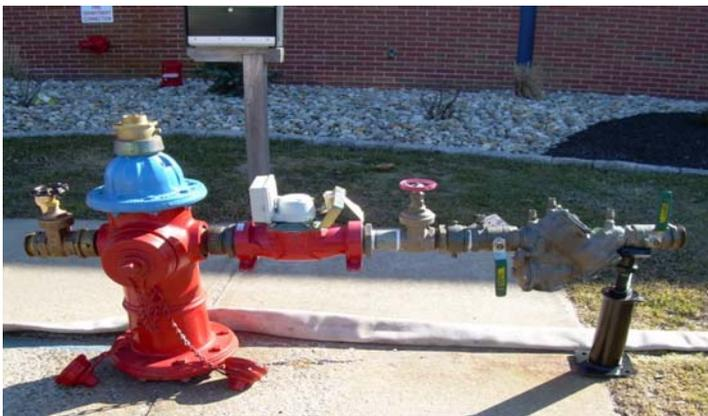
City to hook up to our system and the hydrant will have a meter and backflow prevention device in place to protect our drinking water system from contaminants (below is a typical installation).
