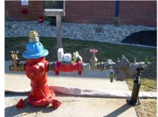
from our system will have trained personnel authorized by the City to hook up to our system and the hydrant will have a meter and backflow prevention device in place to protect our drinking water system from contaminants (pictured to the left is a typical installation).
